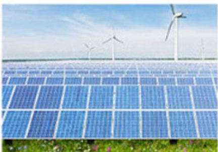
SOLAR PHOTOVOLTAIC POWER SUPPLY
